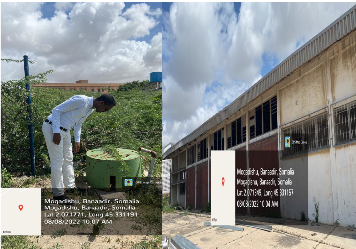
Site 1: Well in IVTC Center (needs to be upgraded)
